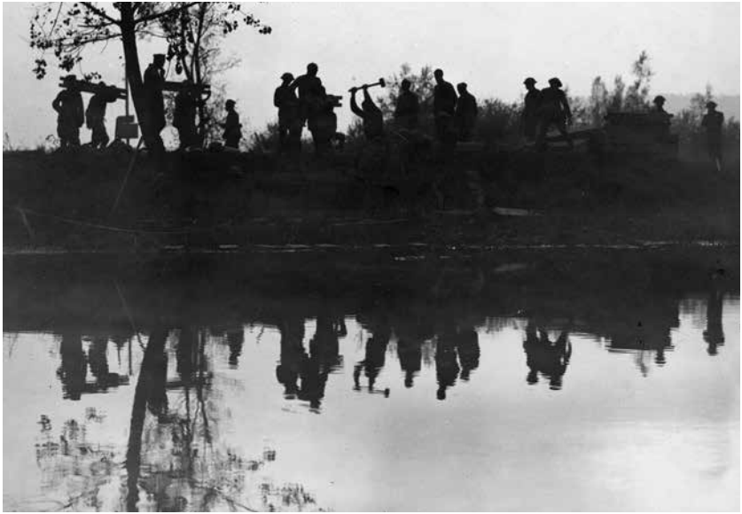
Engineers repairing a road at dusk (National Archives)
